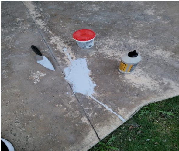
Minor pool area repairs
