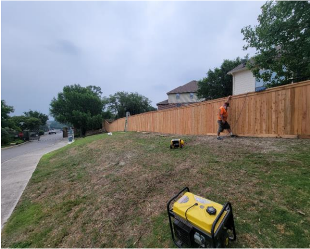
Coves Fence Work
