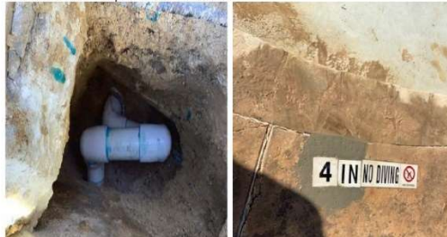
Pictures After Repairs Were Made
