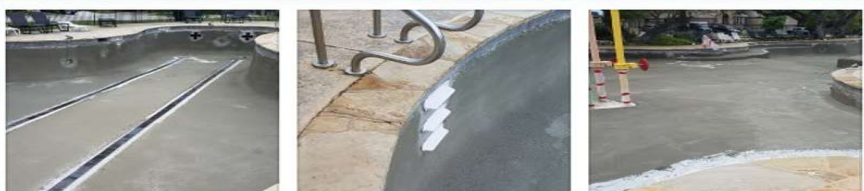
New steps throughout and first layer of plaster cement:
